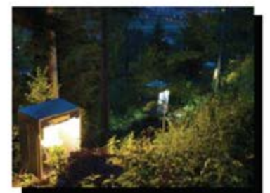
Light sources with a CCT of 3000K or 4000K and a spectrum only providing visible light have proven to be most environmentally friendly solutions
