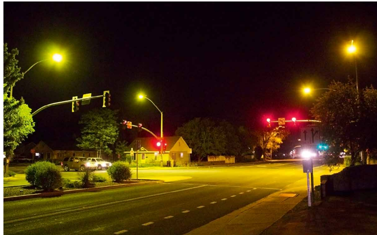
Figure 3: Filtered LED (left) and phosphor-converted amber LED (right) are shown here in a test installation at an intersection in Flagstaff, Arizona. The City of Flagstaff is currently testing these and other low-blue-light LED technologies for the replacement of its existing sodium municipal lighting system (credit: IDA / John Barentine)
