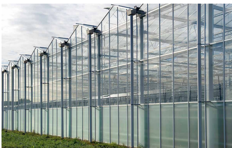
Figure 2: Example for a Venlo style greenhouse
