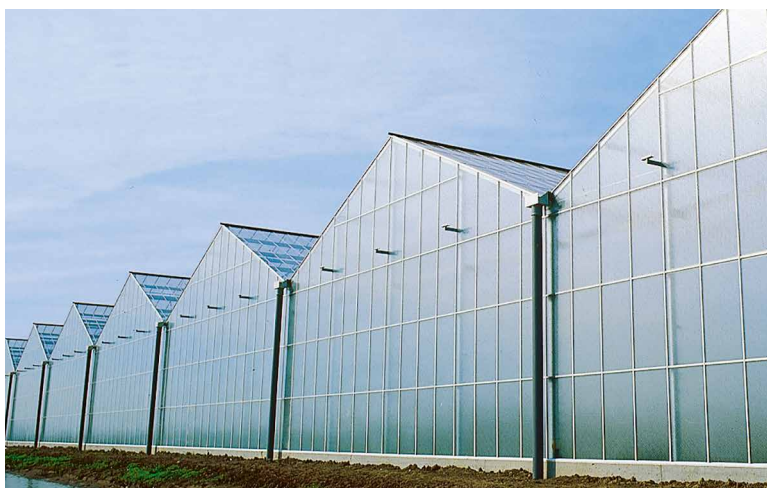
Figure 3: Example for a wide span greenhouse
