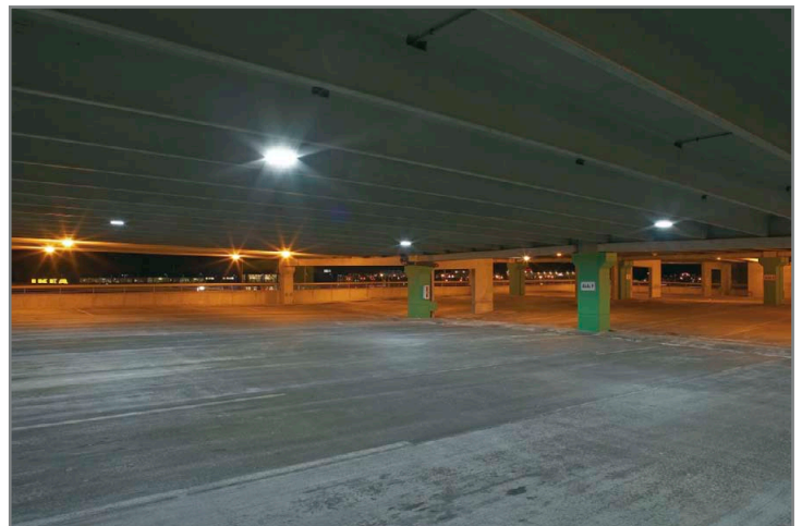
Parking ramp with Beta LED luminaires
