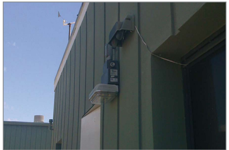
Figure 5: The SafeSite® is a new generation of industrial lighting fixture, which uses LED technology.
