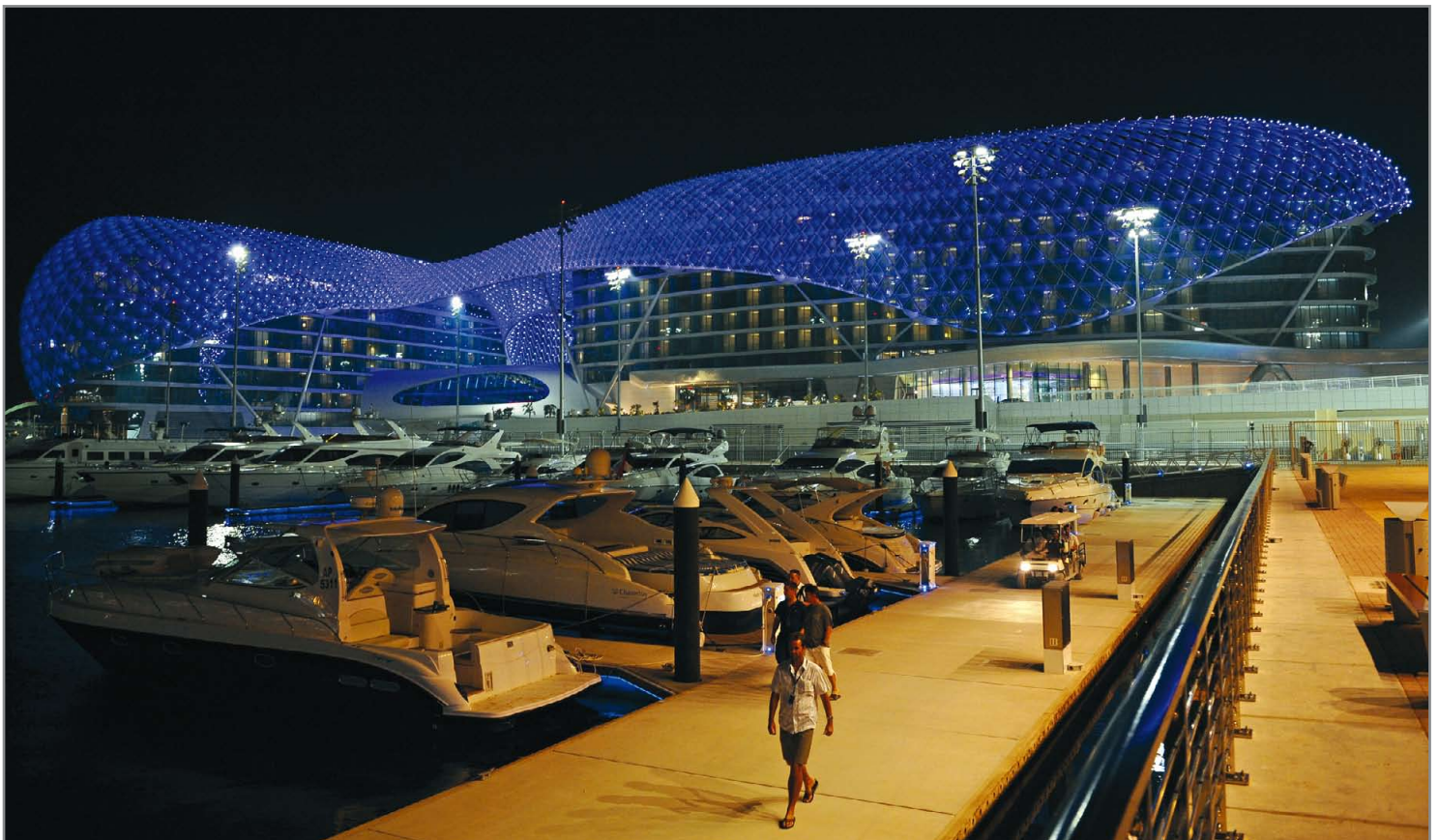
A total of 208,800 LEDs were used on the project making it one of the largest LED projects in the world.
