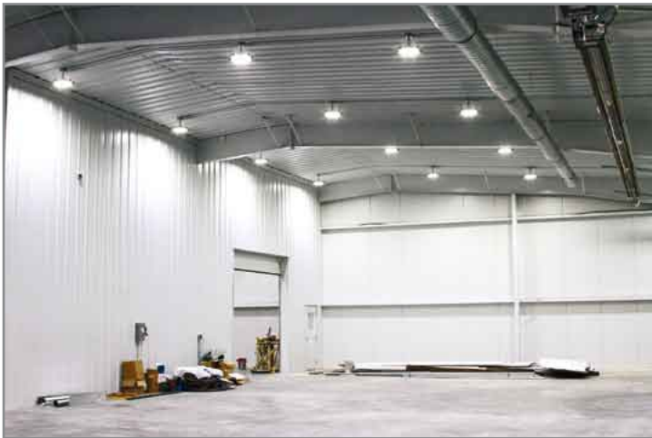
Figure 1: Frontline's new processing facility with LED High Bays from 7 metre high ceiling.
