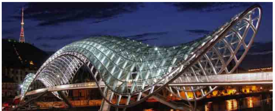
The modern bridge with its dancing white lights forms a striking contrast with the historic buildings in this capital city of 1.5 million
