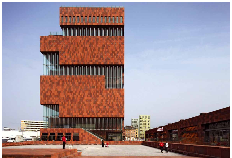
MAS is the first museum in Benelux which is completely fitted out with LED lighting
