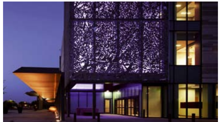
Narrow beam optics with light diffusing film were used, and half of the fixtures were precisely focused to direct light onto the vertical fabric planes*
