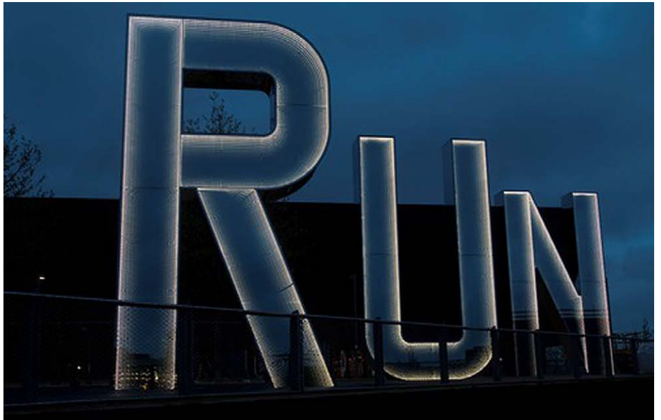
A total of 8464 high-power LEDs make the lighting installation shine at night
