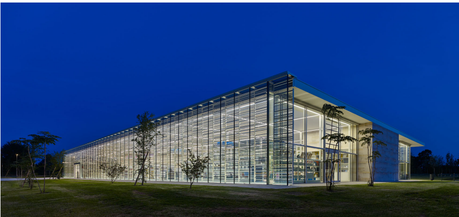
Performance iN Lighting project: MEDIATHEQUE LES 7 LIEUX - Bayeux - France.
