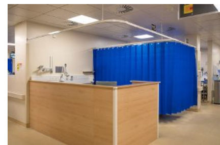
BIOLUX HCL products from Ledvance provide biologically optimized day-night lighting that reflects natural circadian rhythms, to improve sleep, concentration and mood
