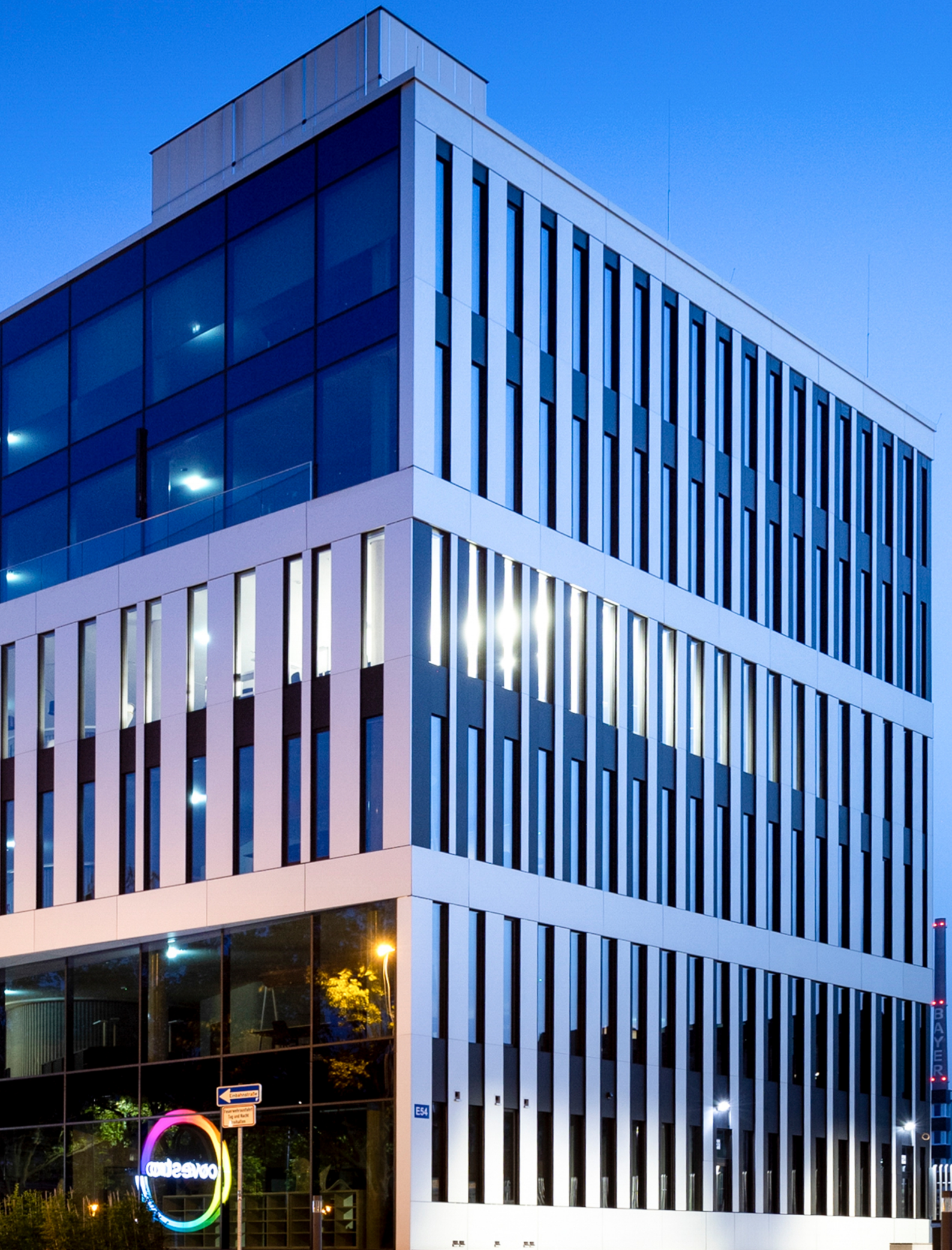
Covestro Headquarters constructed of two-story modules with facade setbacks.
