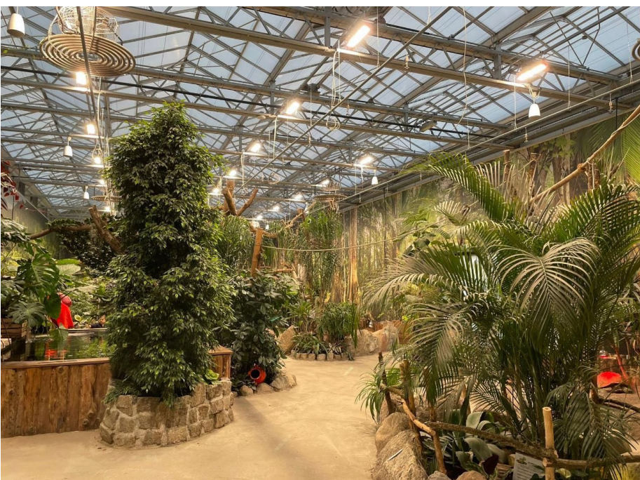
Figure 6: Modular lighting system for plant optimization from Engel Lighting in practical use. (Source: Engel Lighting)
