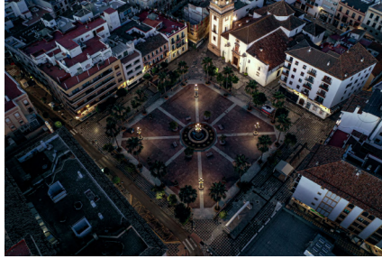
Figure 8: Lighting renewal project in Algeciras, Signify.
